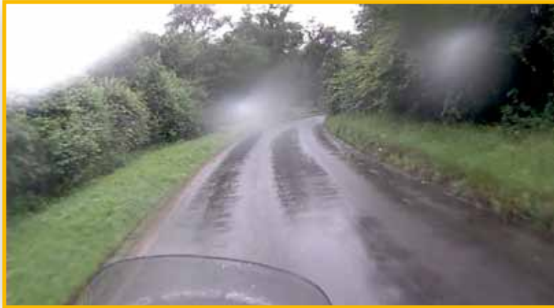
This photo shows polished areas of the wheel tracks.
